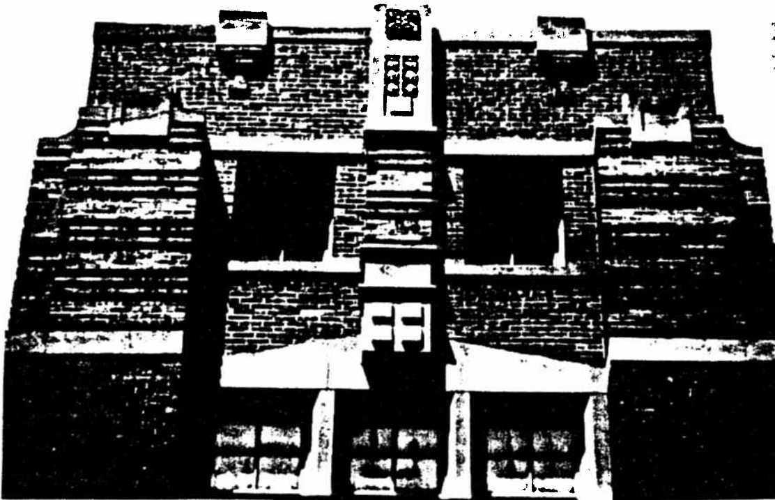
The elaborate details of the building's main tower suggest anthropomorphic facial features.
